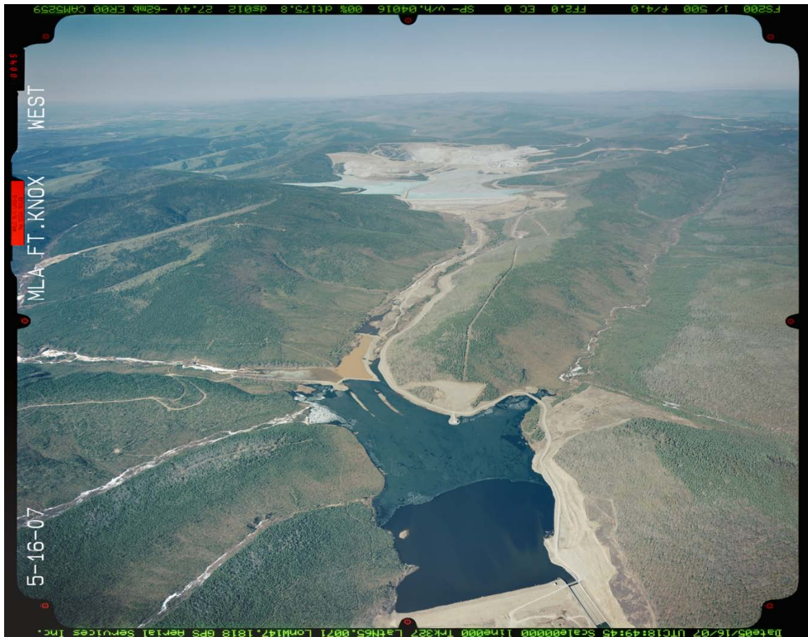
Figure 1. Aerial photograph provided by FGMI – water supply reservoir in lower part of photo and the tailing dam and impoundment in the upper Fish Creek valley.
